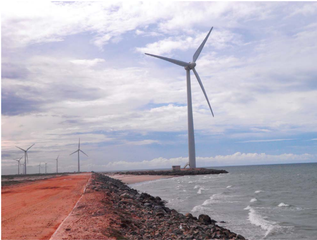
Fig. 5. Wind turbine in Acaraú requiring protection from coastal erosion. Source: Caroline Loureiro.
