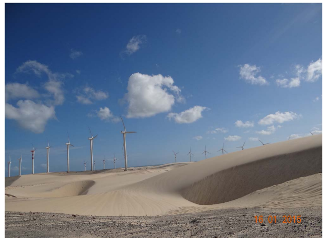
Fig. 4. Wind farm in Xavier constructed in dune field. Source: Jocicléa de Sousa Mendes.
