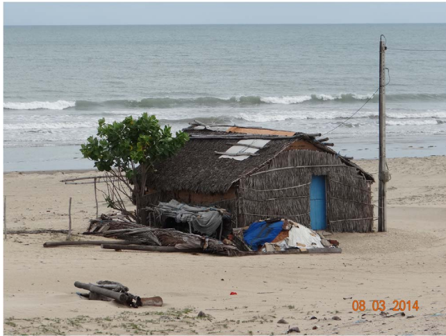
Fig. 6. Wattle-and-daub house in Xavier that was replaced by a brick house funded by mitigation policies. The electricity connection was established after construction of the wind farm.
